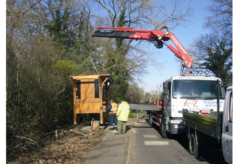
A typical delivery with a crane lorry
